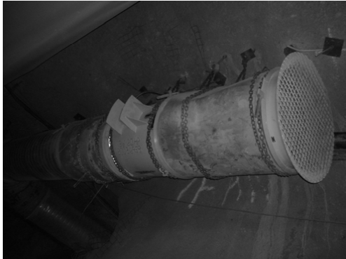
Figure 2. 112 kW fan c/w 1220mm Ø Duct
