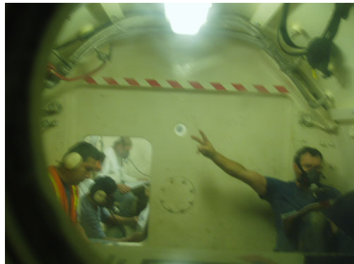
Figure 4 – Workers during oxygen decompression. (Notice the technician without a B.I.B.S mask within the airlock assisting workers during decompression.)
